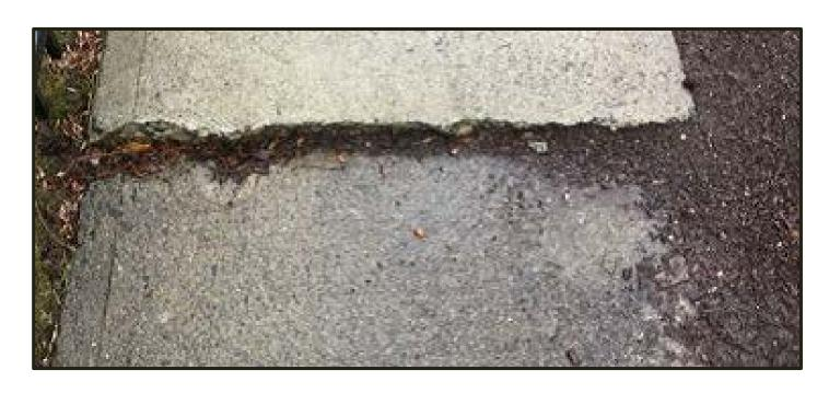
Broken lifting/heaving walkway-Tripping Hazard
