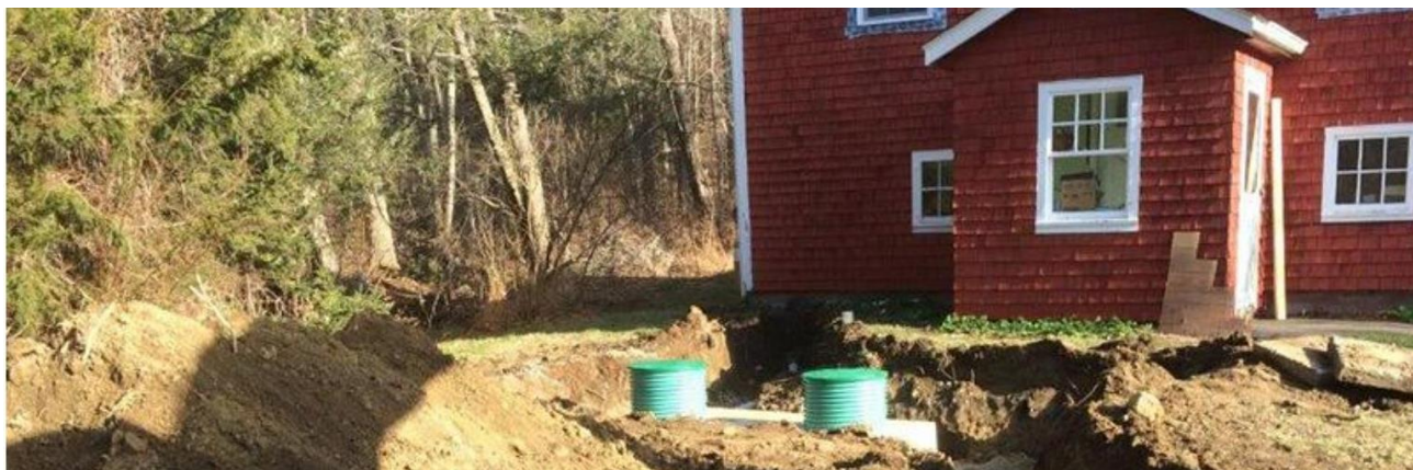
Figure 3-3. Onsite Wastewater Treatment Systems Example from RIDEM
