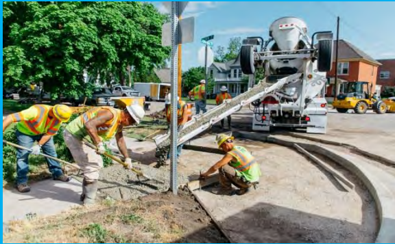
1. Improved sidewalks and crossings
