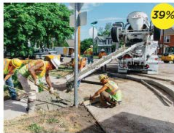
Improved Sidewalks and Crossings
