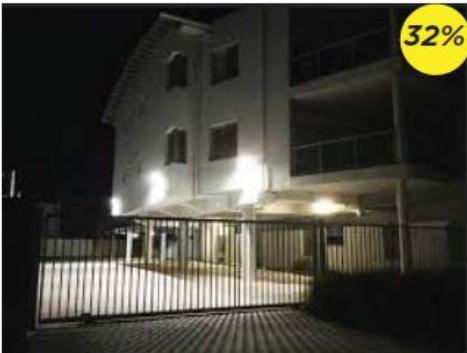
Security and Lighting
