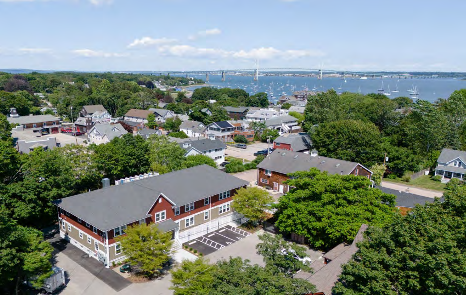
2 Hammett Court in Jamestown provides 12 affordable and accessible apartments for individuals and families, including those with physical or intellectual and developmental disabilities. This innovative project — a partnership between Looking Upwards and SWAP — involved the adaptive reuse of an existing commercial building.
